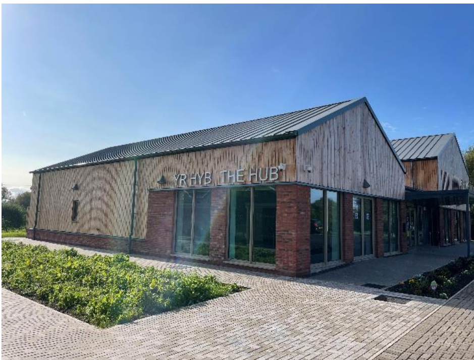
Image of Magor Community Hub partly funded via significant s106 agreement financial contributions from local developments allocated in the Local Development Plan (above); and the building as constructed in September 2023 (below).
